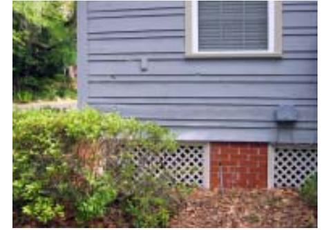
*Wood lattice infill with brick pier.*
