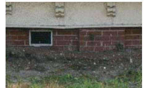
*Enclosing a pier foundation with continuous infill is not recommended.*
