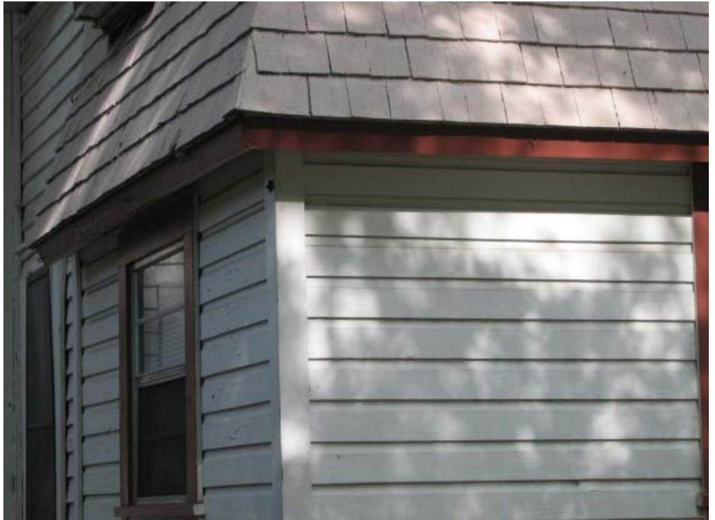
*The exterior fabric of this house in the University Heights North District has both wood shingles and horizontal wood siding.*
