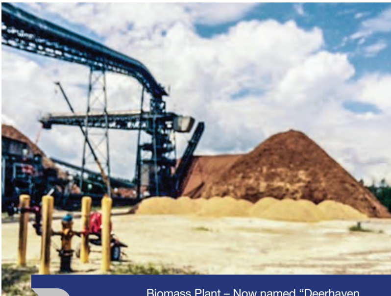
Biomass Plant – Now named “Deerhaven Renewables”
