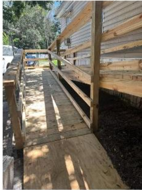
Wheelchair Ramp – Mr. Robert Goetz
