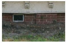
Enclosing a pier foundation with continuous infill is not recommended.
