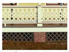
Lattice infill at pier foundation with pier expressed.
