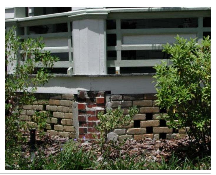
Foundation repairs, the historic materials should be retained, repaired as needed, or replaced with similar materials.
