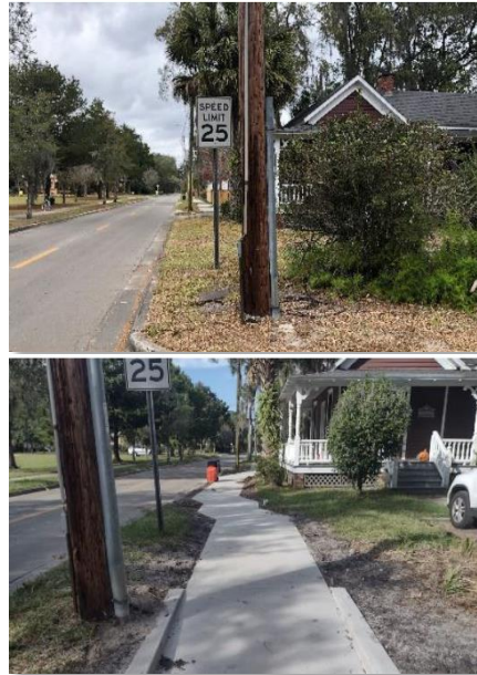
NE 7 th St Sidewalk (Before & After)
