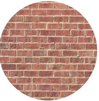
Revitalized Existing Brick
