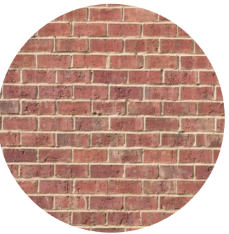
Revitalized Existing Brick
