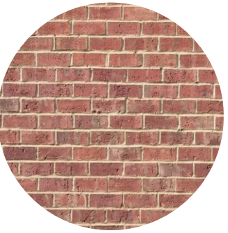
Revitalized Existing Brick
