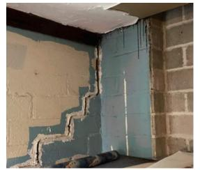
Cracking and Tar Roofing Leaking into Multipurpose Wing
