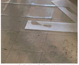
Pooling Water, Roof Leak, Multipurpose Wing
